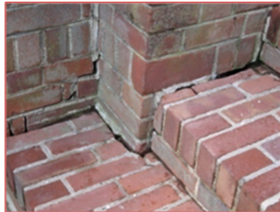
Serious brick joint failures
