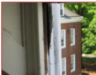
Rotting Wood Frames Inside...
