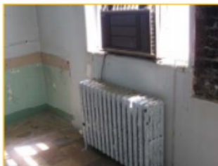
Steam radiators and Window Air Conditioners provide Heating and Cooling
