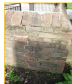
Exterior Brick In Very Bad Condition
