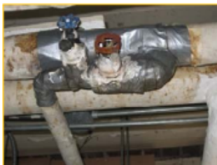
HVAC System kept Operational With Duct Tape
