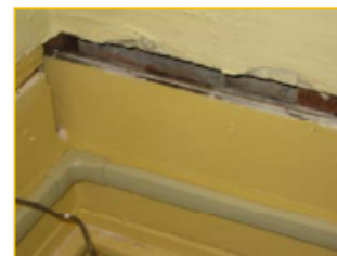
Plaster Delaminating
