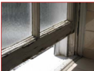
Rotting Single Pane Windows are Energy Inefficient
