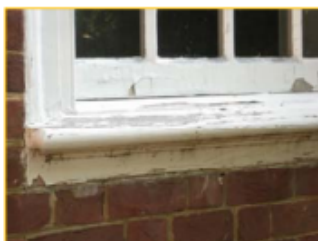
Major Effort Needed to Repair Exterior Wood Surfaces
