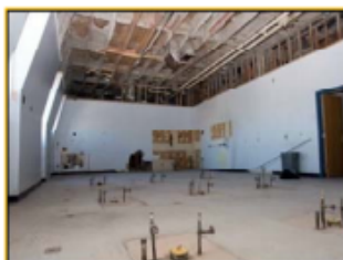
Failed Roof Structure Required Shutting Down and Relocation of Active Research lab
