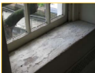
Interior Finishes in Disrepair, lead based paint
